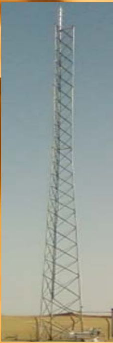
Sample Structure For Master & Repeater RTUs
