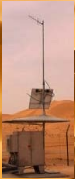
Sample Structure For Remote RTUs
